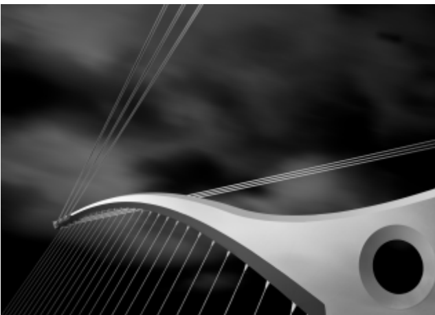
PSSA HM Mark Taylor, Essence of Beckett Bridge, Ireland
