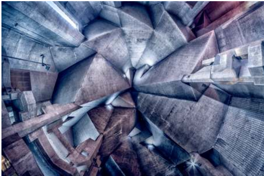
DIPA Mention PDF Barbara Schmidt, Germany, church ceiling concrete
